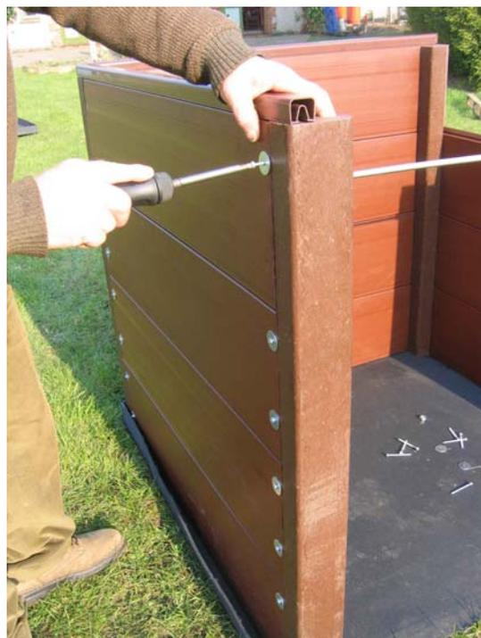
Screwing the base section on
