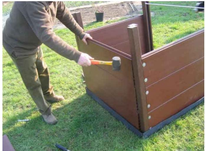
The top plank on the side panels can also be attached now
