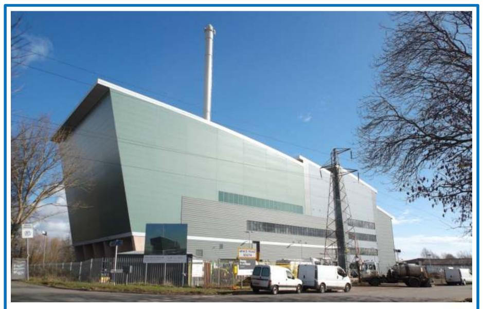
Much of Devon's rubbish is now taken to an 'Energy from Waste' plant where it is incinerated to generate electricity.
