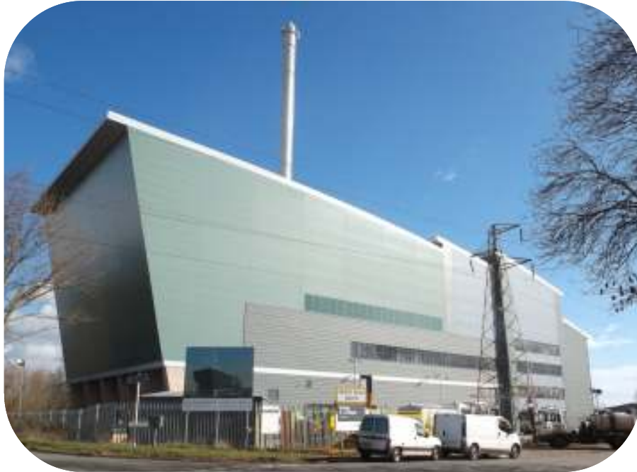
Energy from Waste plant
