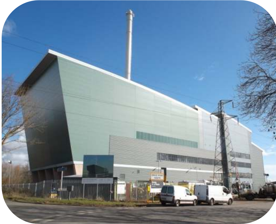
Energy from Waste plant
